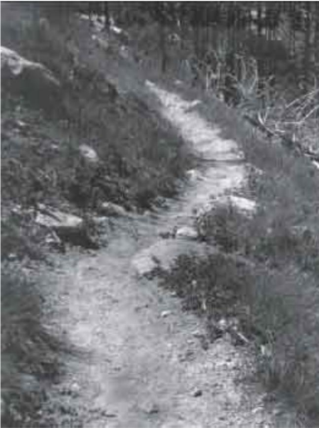
**Figure 3 - Rocks and logs help to keep the trail in place. Remember, this is a path through nature, not a monument to Attila the Hun.**
